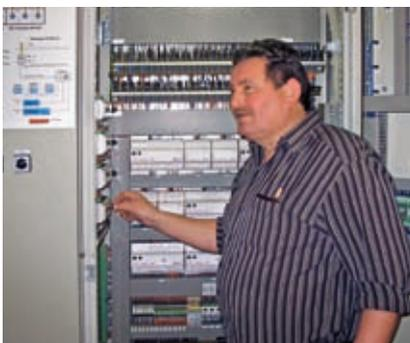
Reinhold Buschle adjusts the  $\dot{V}_{MIN}$  and  $\dot{V}_{MAX}$  parameters of the VAV controllers on the Fan Optimiser.
